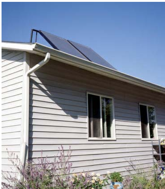
Tilt-mounted solar hot water panels
